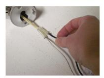
**6.** Turn on power to ensure light is working properly. Note: LEDs are polarity sensitive. If the handle does not light try reversing the connections. Push the wiring into the wall and re-attach handle.
